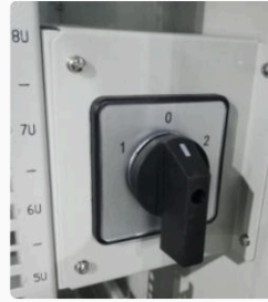
125A power source switch
